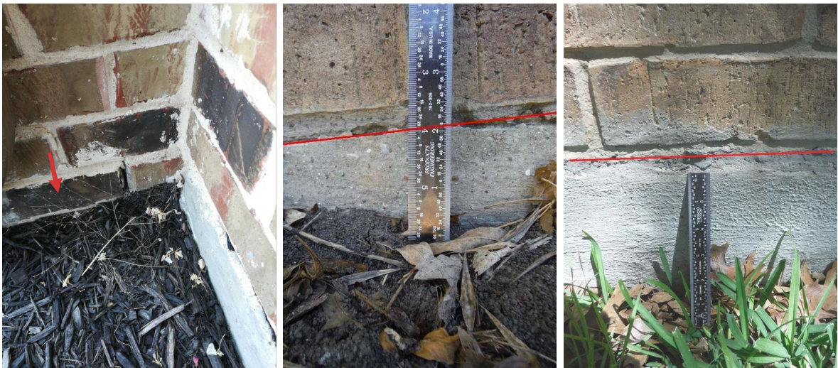
Insufficient Clearance to brickledge 2" (EXAMPLE) Sufficient clearance to brickledge 6"+ (example)
