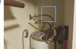
4.1.3 Water Heating System **NO DRAIN PAN OR PIPE**
