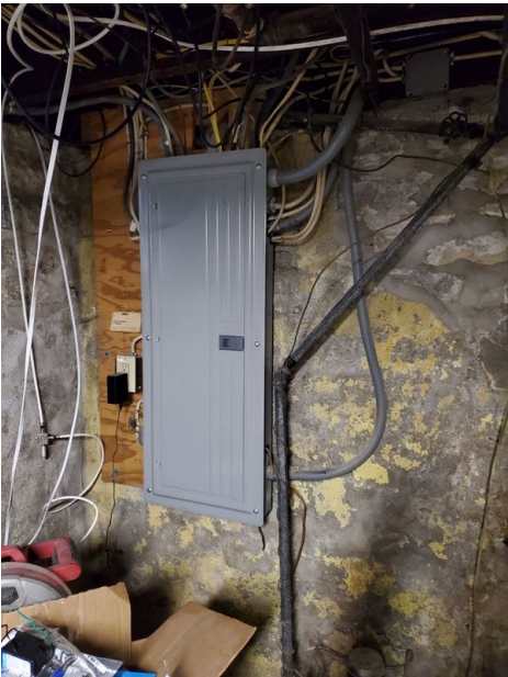
Main Shutoffs: Electrical Disconnect Basement
