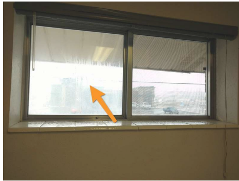
Moisture inside of the window.
