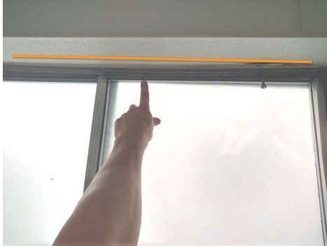
Top of window frame has bowed down in the first floor south bathroom.
