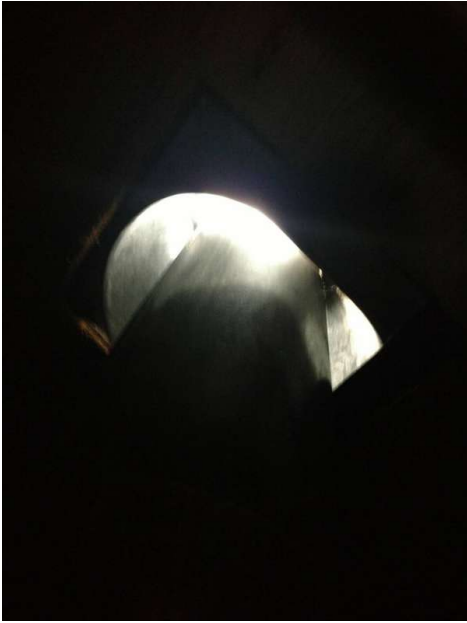
Daylight coming in from around vent pipe.
