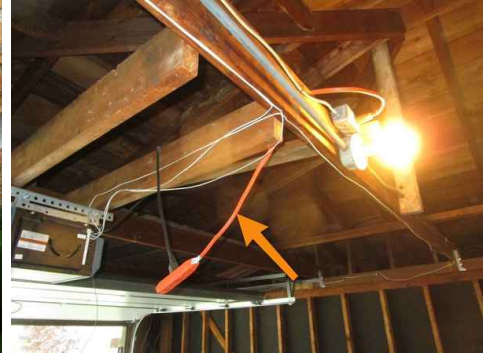
Extension cored wiring - garage
