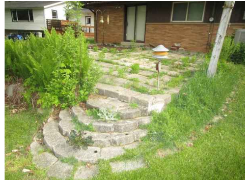
Improper and damaged steps and no handrail
