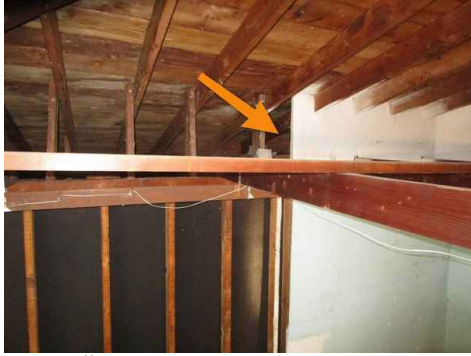
Firewall missing
