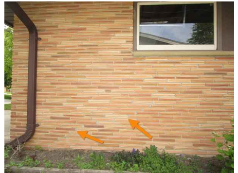
Cracks at NW corner of garage - may be related to movement (though not confirmed)
