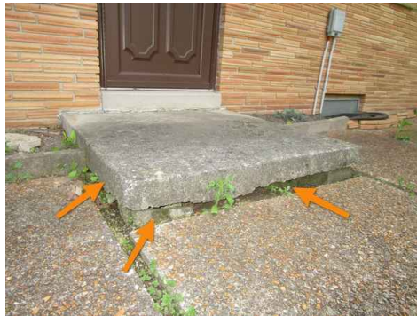
West stoop - Gaps and deterioration
