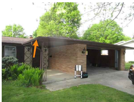
Improper pitch and ponding
