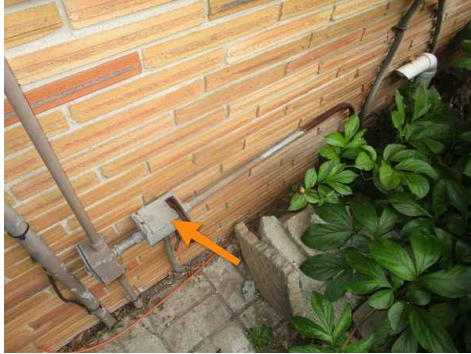
Outlet installed face up and closed with clamp - north
