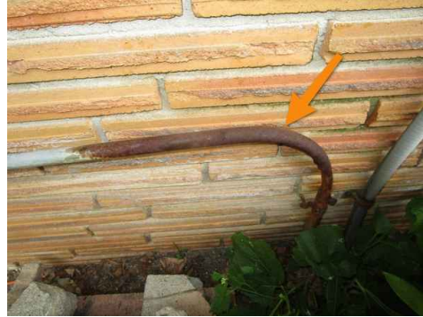
Rusted conduit with leaks/holes in conduit
