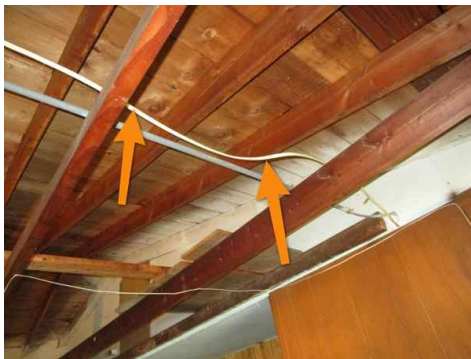
DIY wiring - garage
