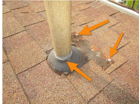
Rusted flashing, exposed fasteners and damaged boot
