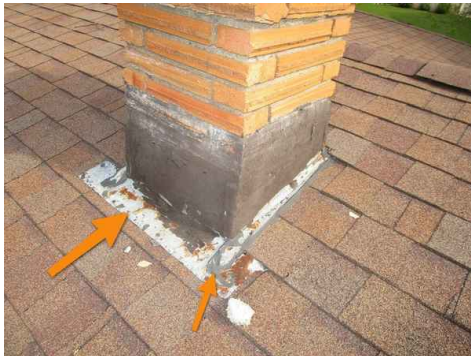
Rust, tarred and improper fasteners
