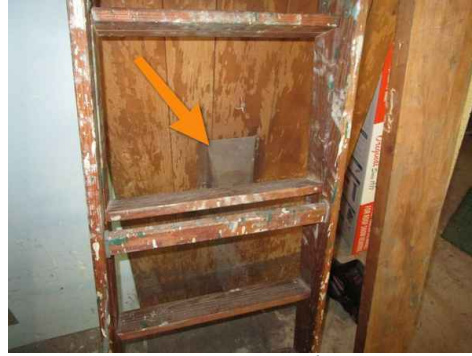
Dryer vent terminates in the garage
