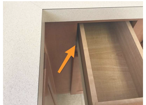
Drawer slide is not attached.
