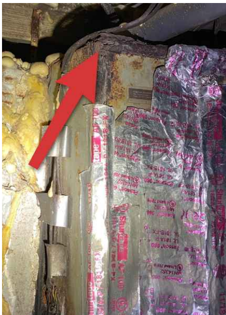
Coil cover rusted and damaged
