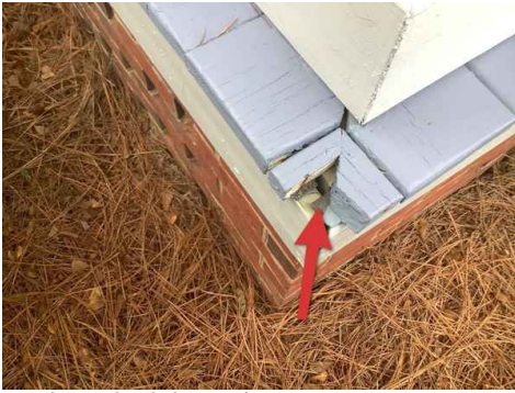
Broken deck board at corner
