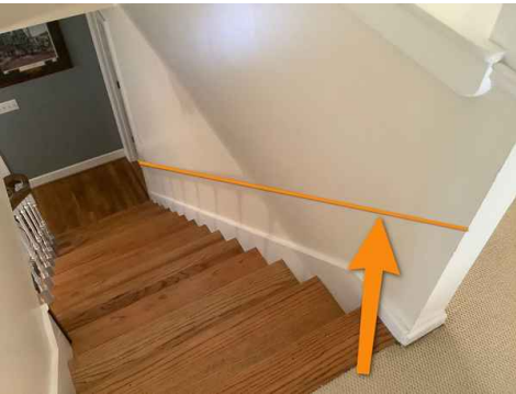
Handrail missing
