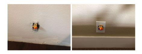
12.11.2 Outlets, Electrical **MISSING COVERS** THROUGHOUT HOME There were missing covers that should be installed Recommendation Contact a qualified handyman.
