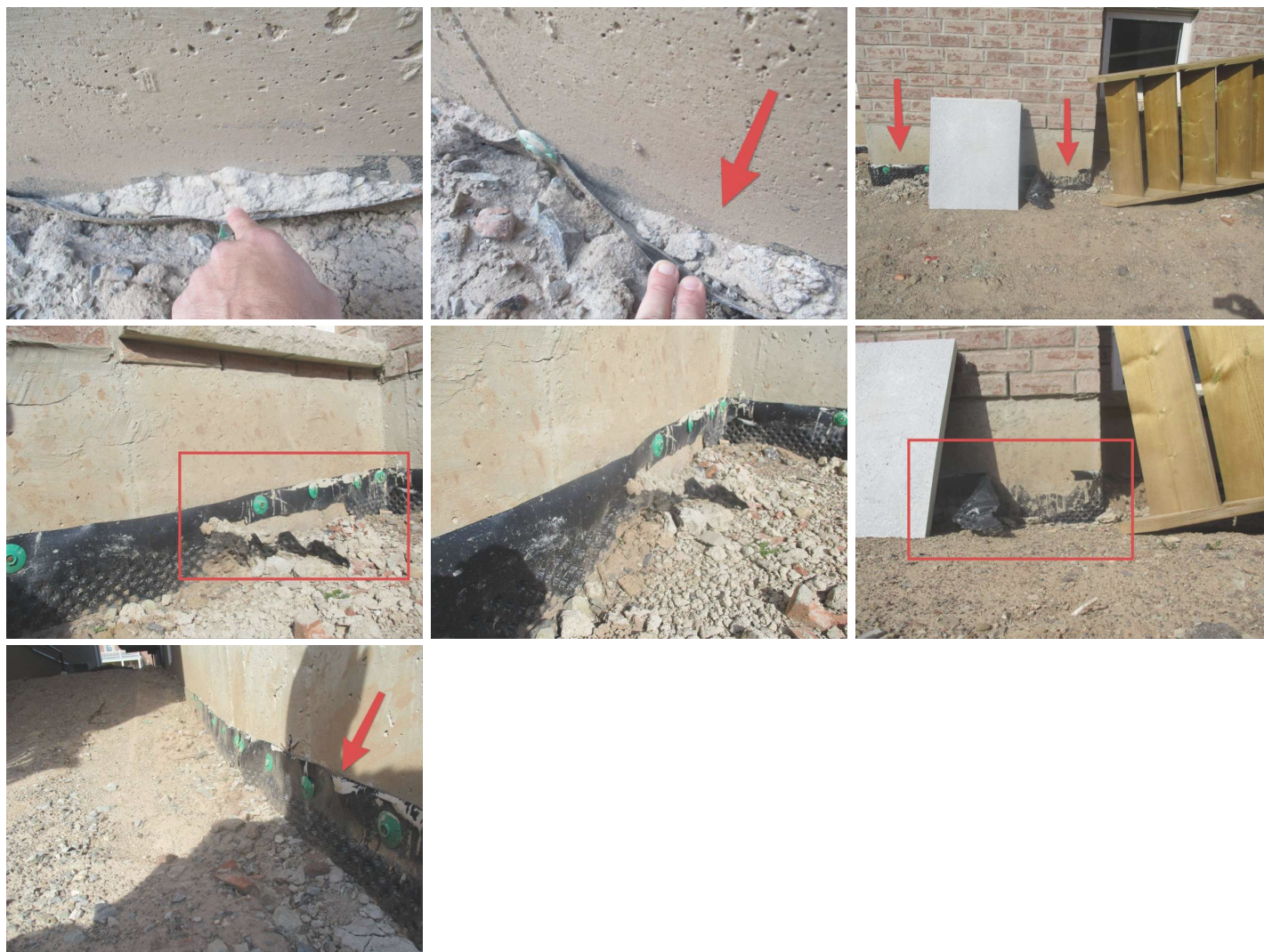
Missing waterproofing sealant
