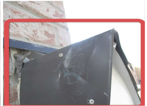
Poor workmanship multiple areas for water penetrations.
