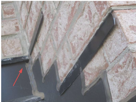
Area for water penetration and pests
