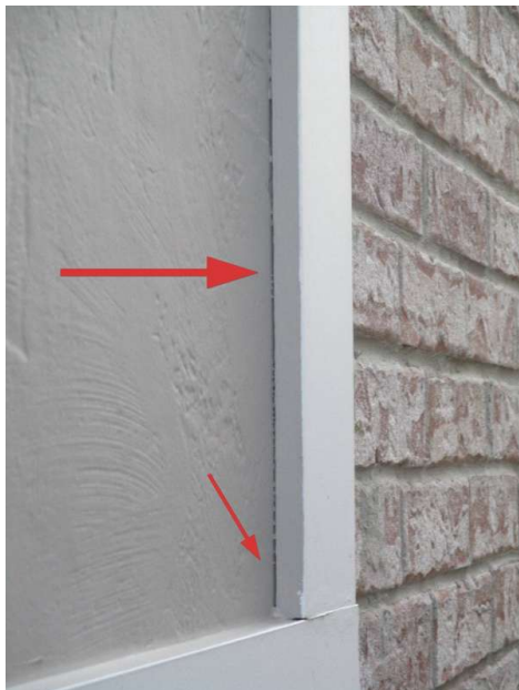
Multiple areas for water penetration and moisture damage.
