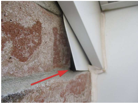
Area for water penetration and pests
