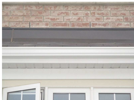
Poor workmanship, missing flashings.
