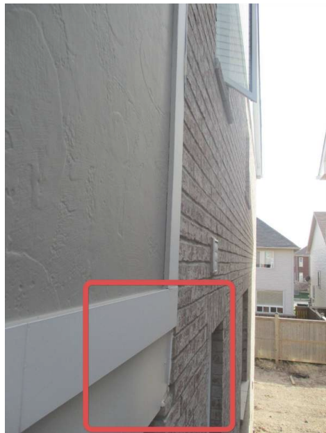
Poor workmanship, missing flashings.
