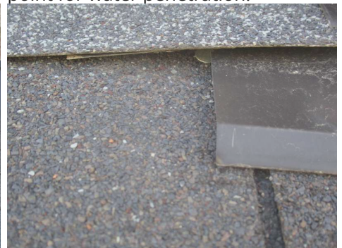
Exposed nails will rust and become point for water penetration.
