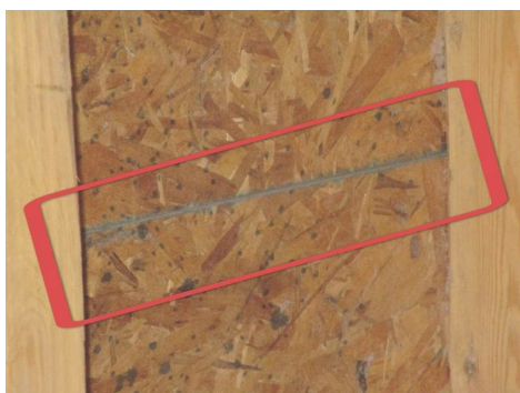
Signs of day light showing at attic cladding areas. Multiple areas of for water penetration and moisture damage. Missing waterproofing membrane, recommend repair or replace.
