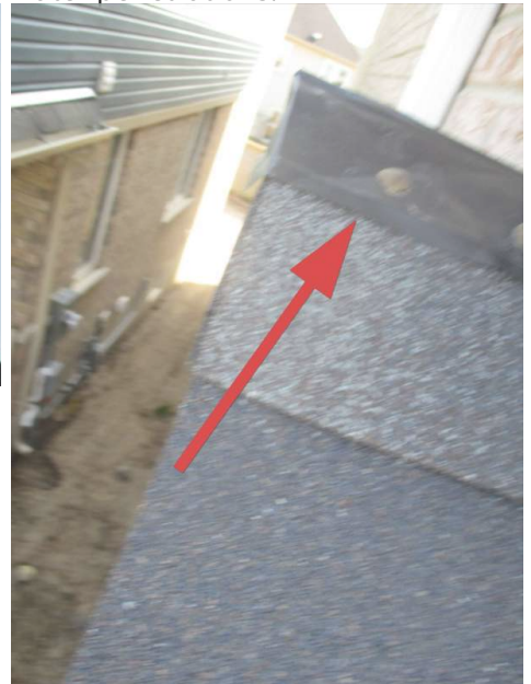
Exposed nails will rust and become point for water penetration.
