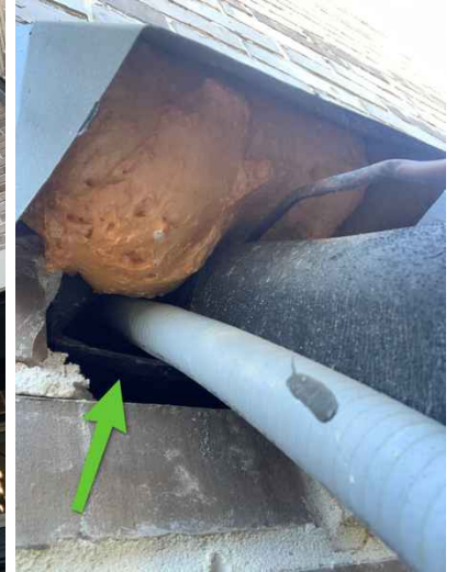
A/C line penetrations into home
