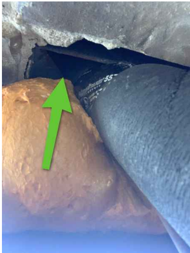
A/C line penetrations into home
