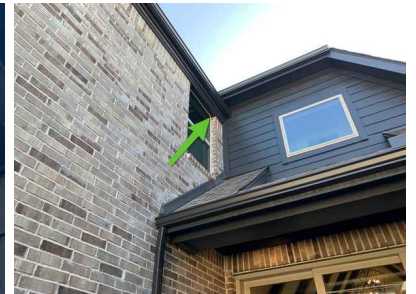
A/C line penetrations into home
