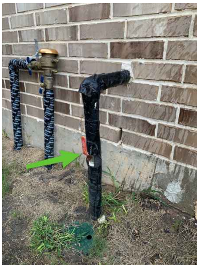
Water Shut-Off Valve
