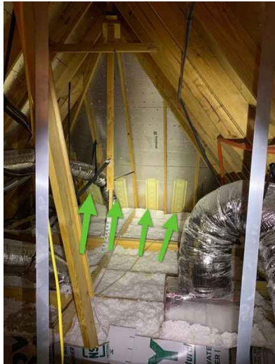
Baffles in attic
