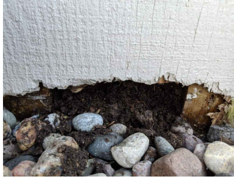
Soil buildup inside wood enclosure
