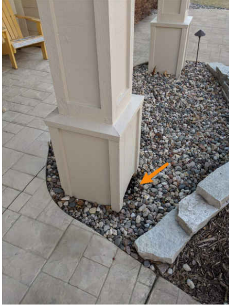
Soil buildup inside wood enclosure
