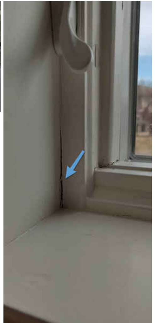
Caulking failed
