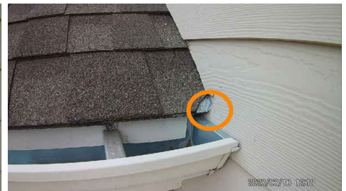
Kick out flashing undersized
