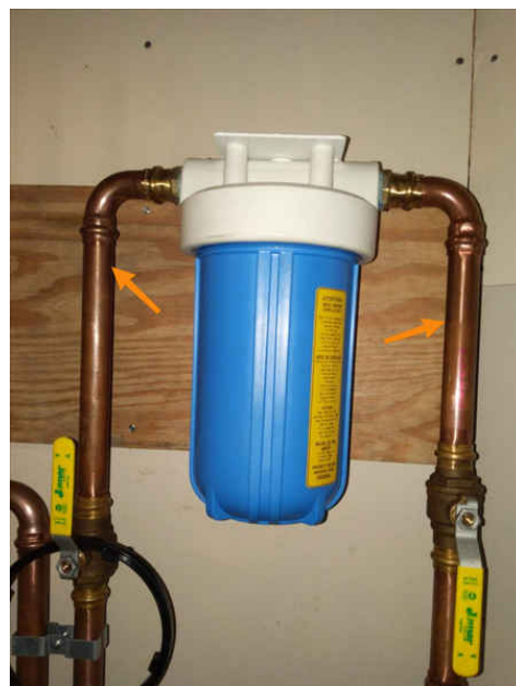
Missing bonding jumper
