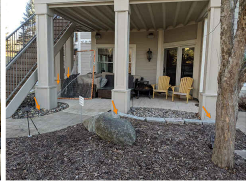
Base of columns at risk for deterioration
