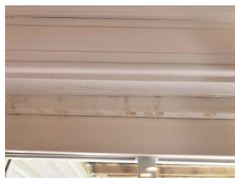
Water spots below ledger in basement
