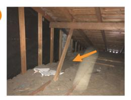
14.5.3 Insulation Notes HATCH MISSING INSULATION
