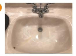
11.1.2 Sink and FaucetSINK STOPPER(S) MISSINGMASTER BEDROOMSink stoppers should be installed if desired.Recommendation
