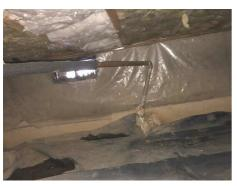
Drain, Waste, & Vent Systems: **Waste pipe Material** ABS
