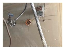
Main Water Shut-Off, **Distribution & Supply: Water Supply Material To House** Copper
