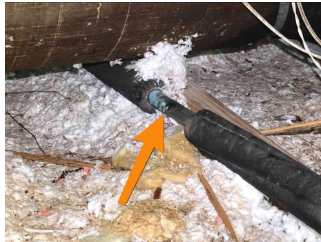
Condensation Inside Attic
