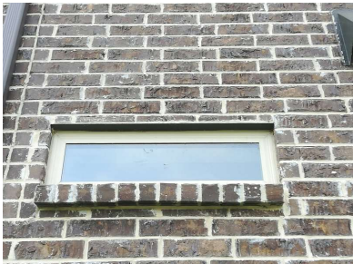
No weep holes installed
