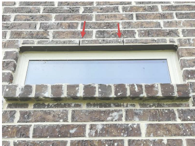
Weep holes installed
