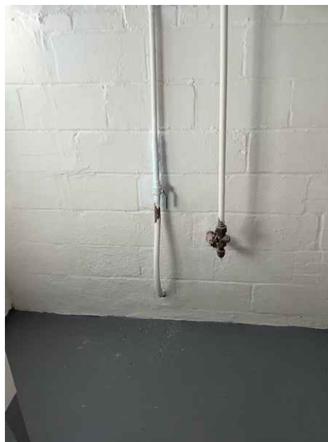
Water and gas shut offs. Laundry room in basement
