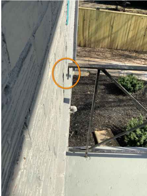
Front door. Rail not connected to house
