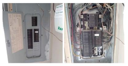
Panel Amperage(s): 200 Amp Service Electrical Panel Manufacture(s): GE
