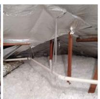
Approximate Insulation Depth: 16-18 inches Type of Insulation Present: Fiberglass
