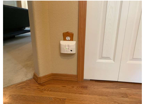
1 of 3 plug-in CO Detectors in the home, 1 on each level
