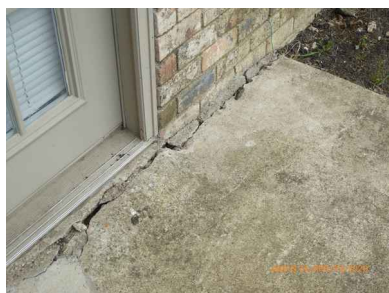
back patio door. Slab separating from patio.
