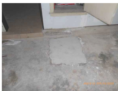
dig spot for foundation repair.
