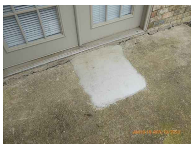
dig spot for foundation repair.
