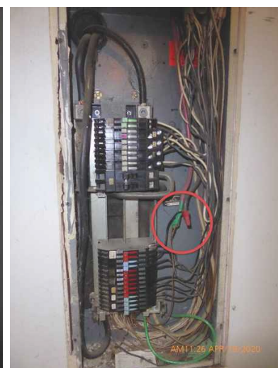
improper connection
