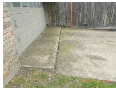
driveway at garage door. Drive separating from garage floor.
