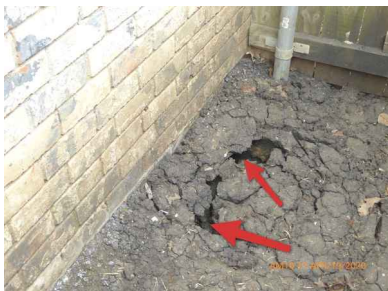
hole is hollow under foundation wall.
