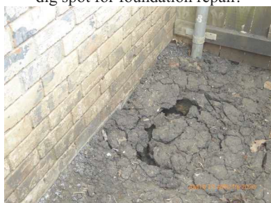
dig spot for foundation repair.
