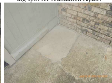
dig spot for foundation repair.
