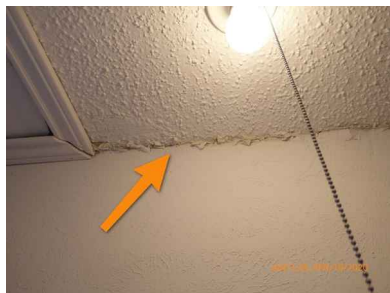
separation from wall and ceiling at north west bedroom.
