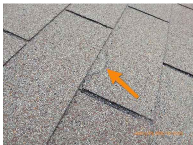
Damaged shingle
