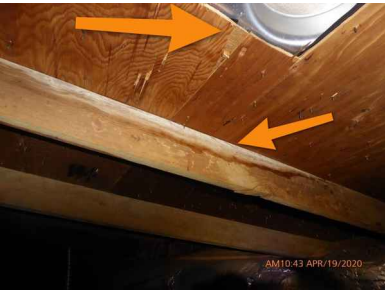
thin brittle sheathing and water damaged rafters.
