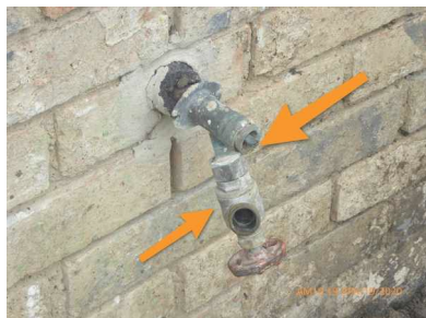
Handle is broken and another valve with a working handle was placed on broken bib.
