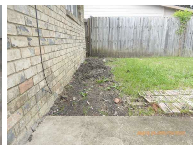
dig spot for foundation repair.
