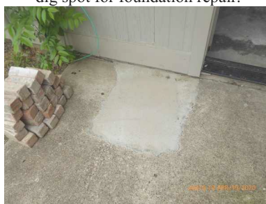
dig spot for foundation repair.
