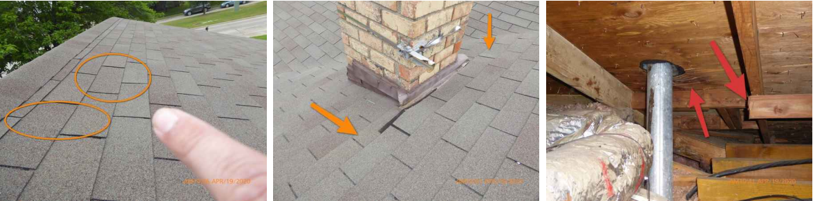
showing rafter support was cut for gas flue pipe clearance. Also shows rotted decking from roof leak.
