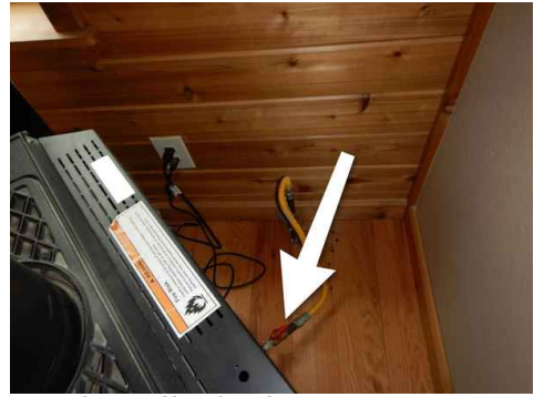
Gas Shut Off Valve for Stove
