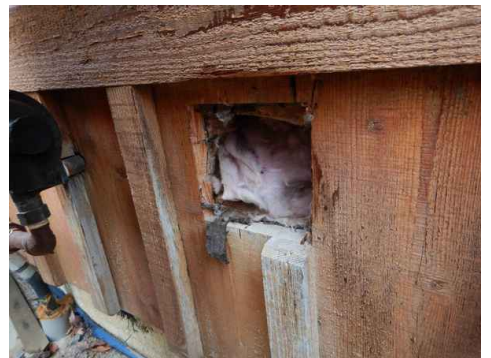
Hole by Gas Regulator
