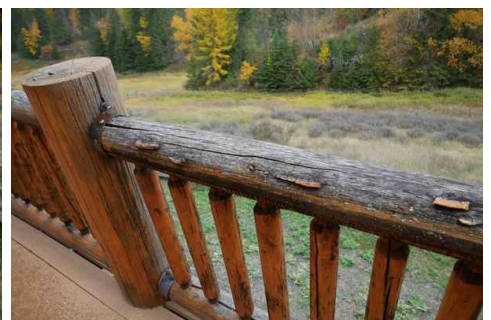
Missing Corner Support Post
