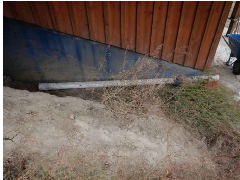
West Side Water Erosion/Mud Slide
