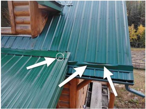
Damage and Popped Screw
