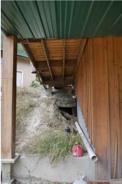
West Side Erosion Under Deck Ramp
