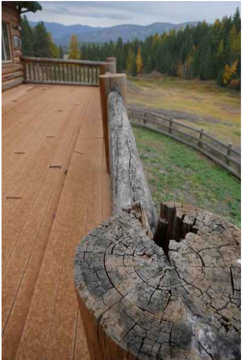
Railings and Posts Rotting and Unsafe
