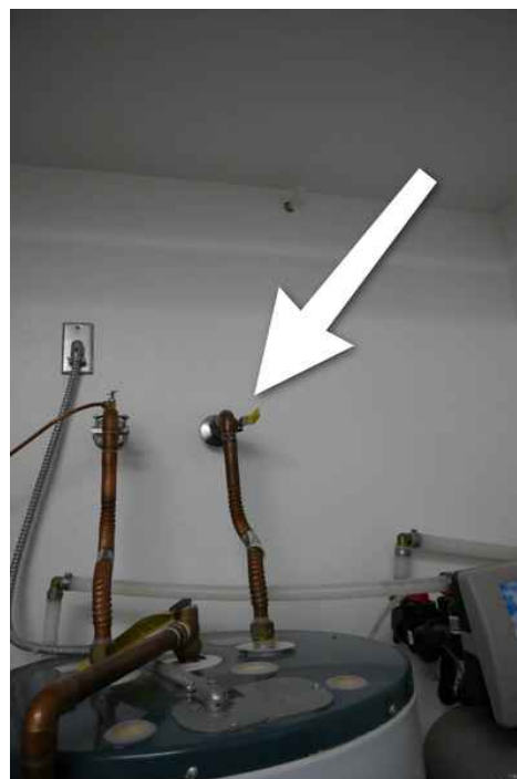
Water Heater Water Shut Off
