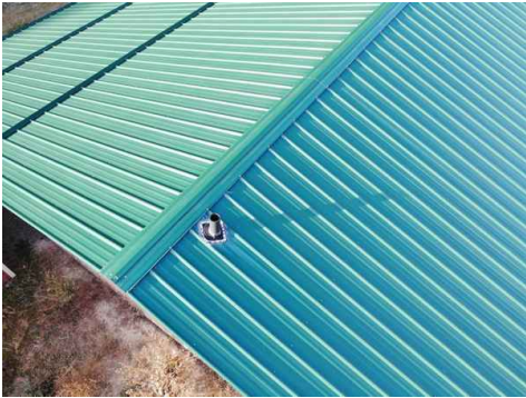
Bathroom Vent Pipe
