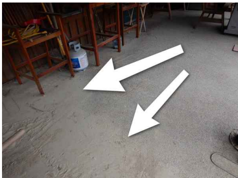
Mud Entering Basement Concrete Area
