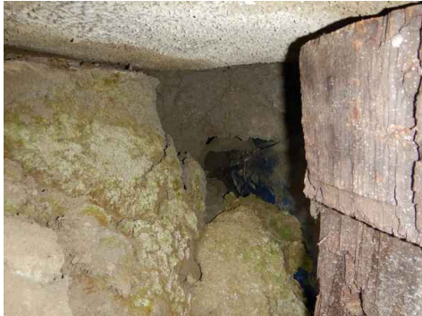
Water Erosion Under the Deck Ramp
