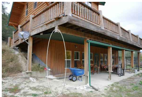
Missing Corner Support Post
