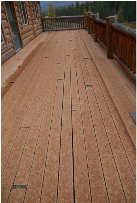
Trex Flooring Unsafe to Walk on
