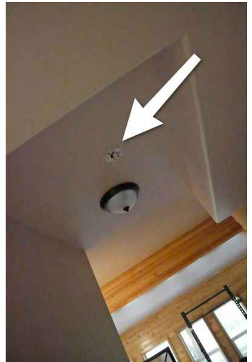
Missing Smoke Detector
