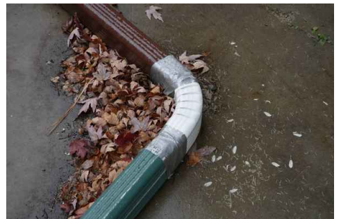
North West Gutter Drain Taped Together
