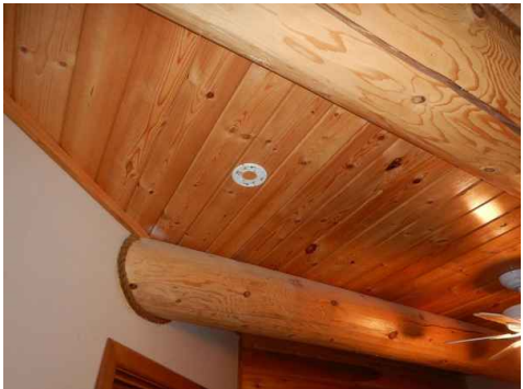
Missing Smoke Detector
