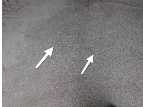
Concrete Cracks
