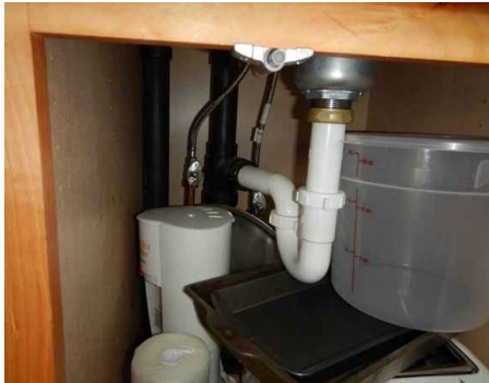
P-trap, Shut Off Valves Under the Sink
