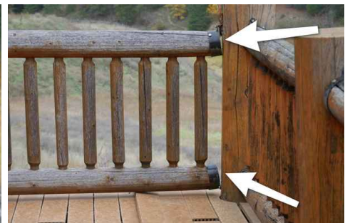
Railing Corners are Detached
