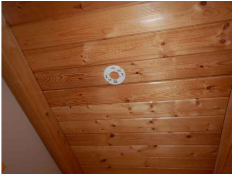
Missing Smoke Detector
