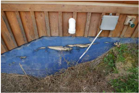
Romex and Cat3 Wires Exposed
