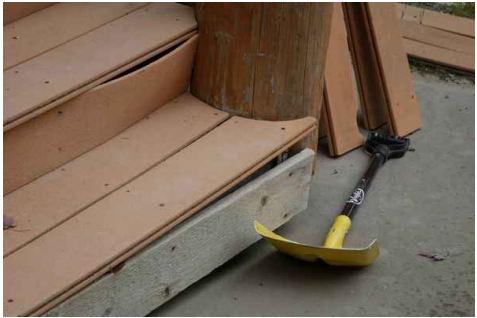
Board Detaching From the Step
