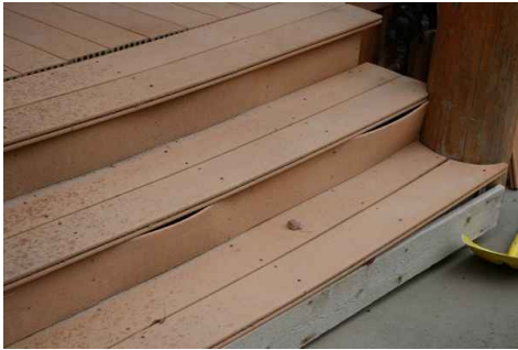
Warped Boards
