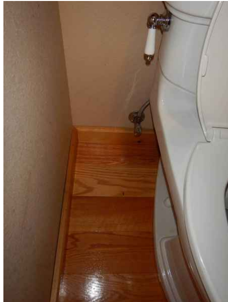
Shut Off Valve by the Toilet
