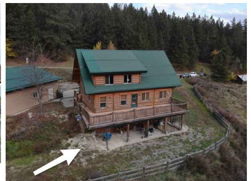
Missing Corner Support Post
