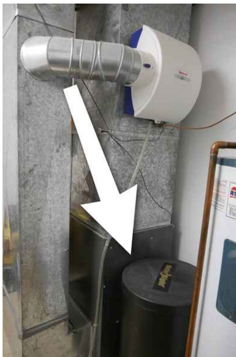
Salt Storage for Water Softener
