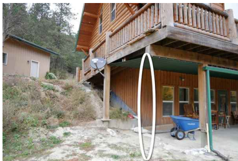
Missing Corner Support Post
