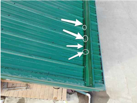
Popped Screws and Damage
