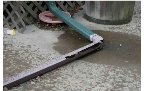
North East Gutter Drain Damaged
