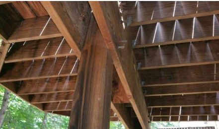
Deck Beam Assembly
