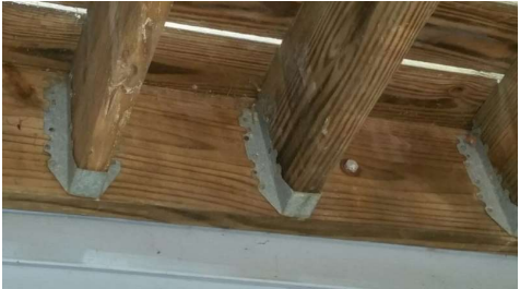
Independent post and beam at the interior side of the deck
